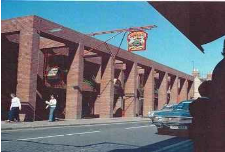
The original High Street colonnade and signage before alterations
